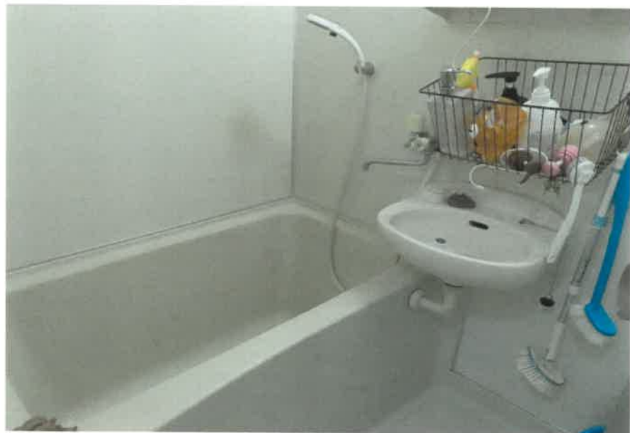
物件2:101浴室の状況
