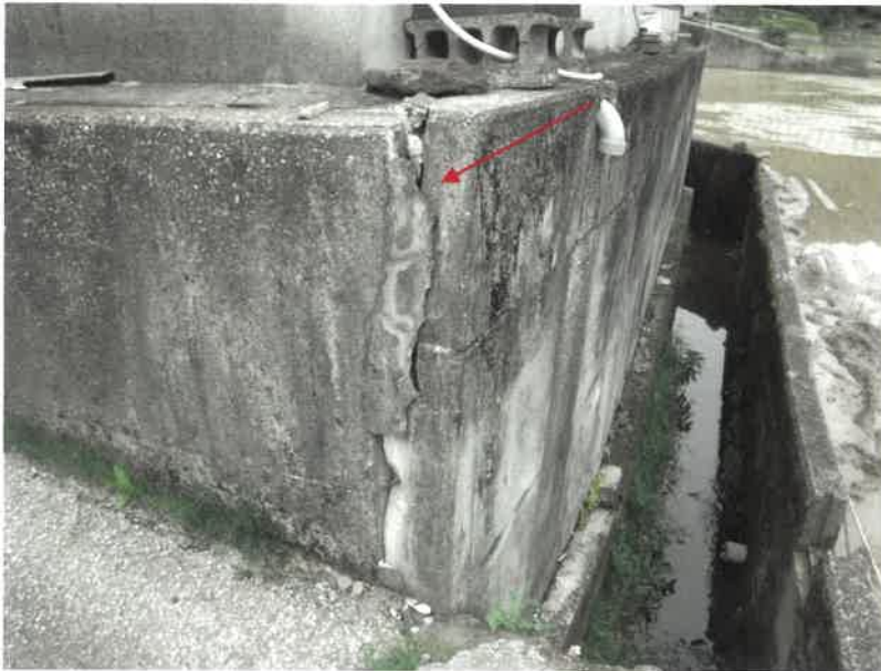
No. 1 物件 1 (擁壁)
